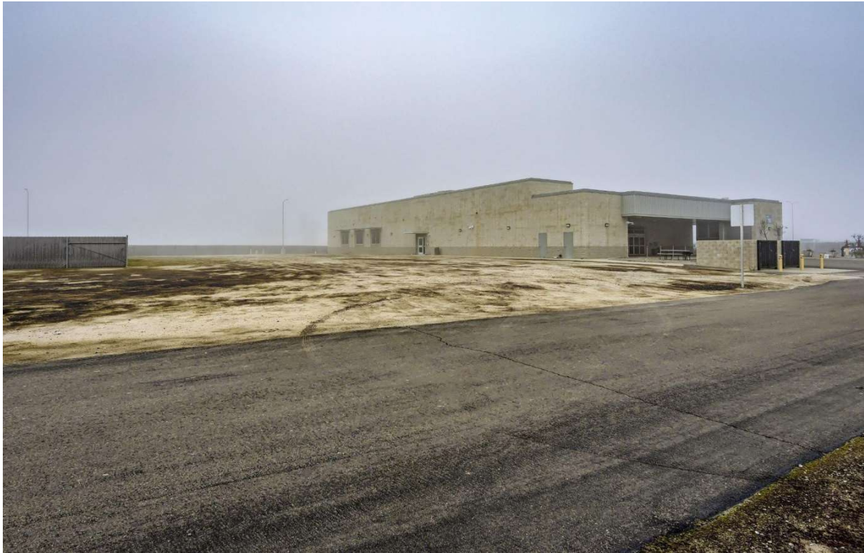
Vacant lot adjacent to the Fresno County Coroner's Building proposed for the future placement of three modular buildings.
